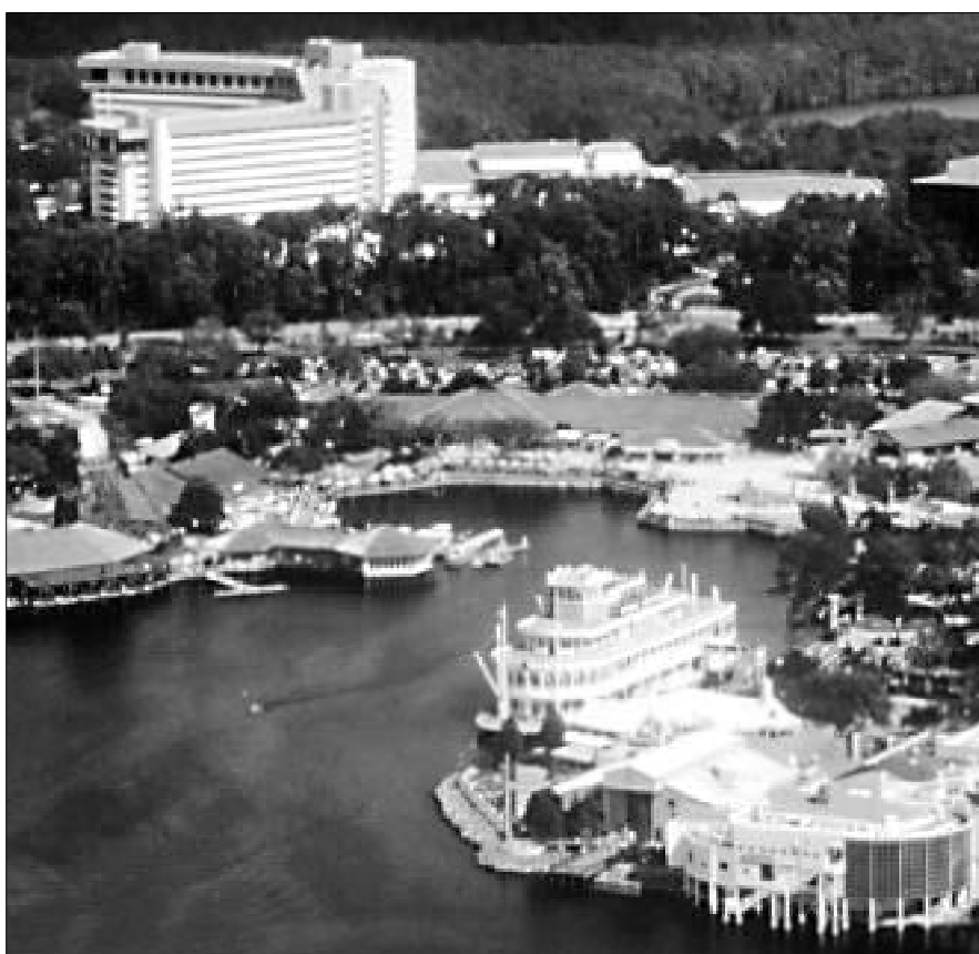
This overhead view of the hotel and its surroundings showcases the beauty of the area and all the amenities available to CALGB Fall Group Meeting attendees.
